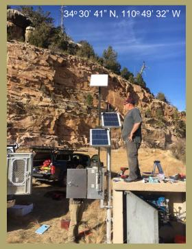
This remote dam, owned and operated by the Arizona Game and Fish Department, had inoperable principal outlet valves and no way to control the actuator remotely. Without a way to monitor lake level and control the principal outlet valves remotely, it was necessary for Department employees to travel several hours to the dam to assess hydrologic conditions and manually actuate the valves.
